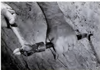
Clean out holes with cold chisel.
